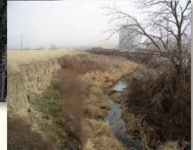
Upstream channel erosion (Pataha Creek)
