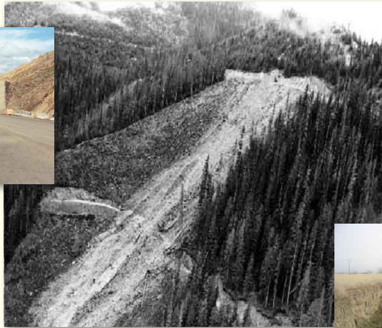
Logging road and landslide (Clearwater National Forest)
