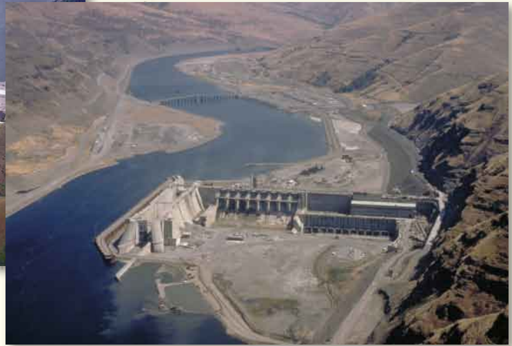
Site Condition During Construction of Lower Granite Dam That May Be Similar to the Breached Condition
