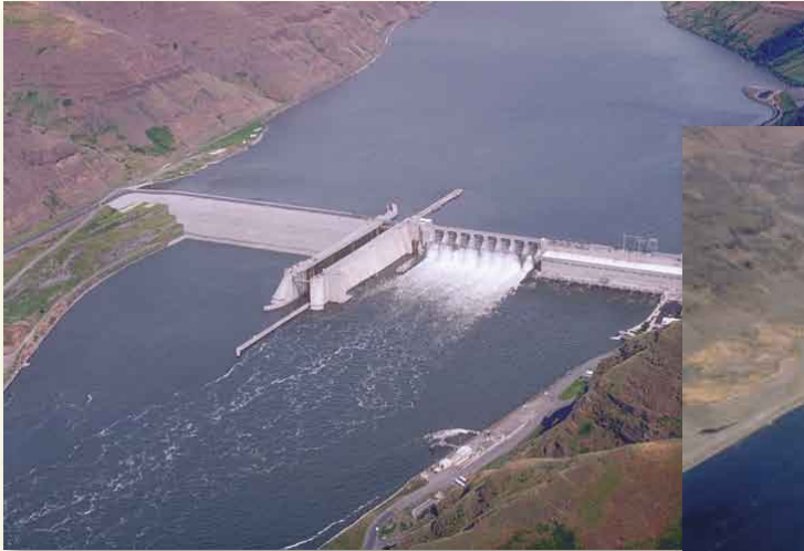
Current Photograph of Lower Granite Dam
